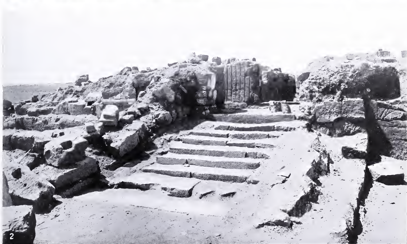
1. View from NE. after excavation, showing the entrance (L).
